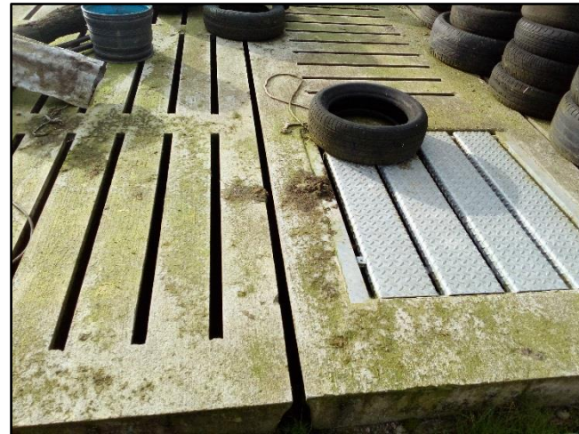
Figure OS4: Slatted Tank
